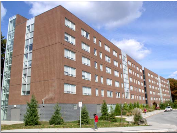
Les Prince Hall, opened in 2006 and one of the first student residences in Canada to be LEED certified, is a LEED silver building. Photo: Janet Woodward
